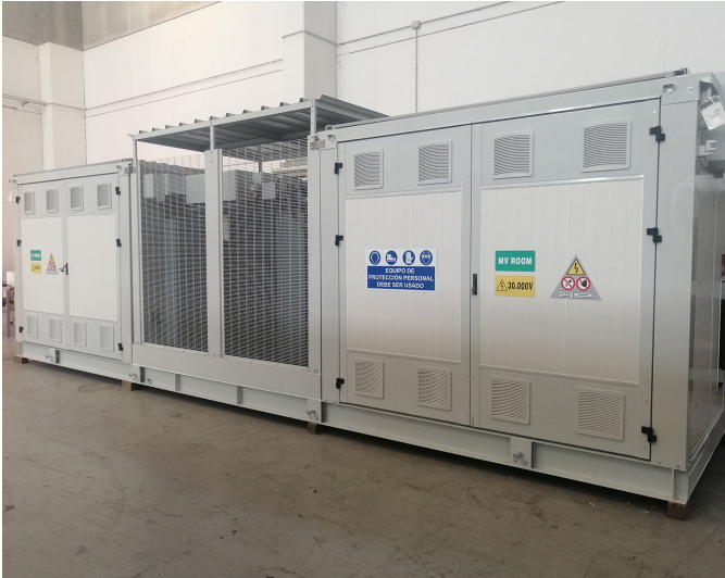
One of the 5000kVA rated/7000kVA peak power SPL transformers filled with FR3 fluid in the solar skid.
